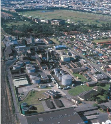
Figure 4. Merebank downstream plant near Durban, South Africa, with an ethyl alcohol production capacity of 40 million litres per year (Source: Illovo Sugar Ltd)
