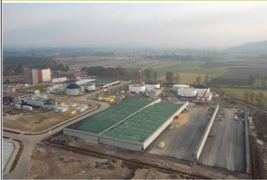
Ariel view of plant
