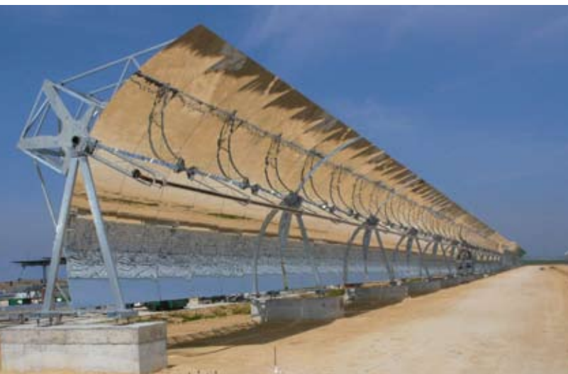
Cylindrical parabolic collectors. Image reproduced with the permission of Abengoa-Solucar.
