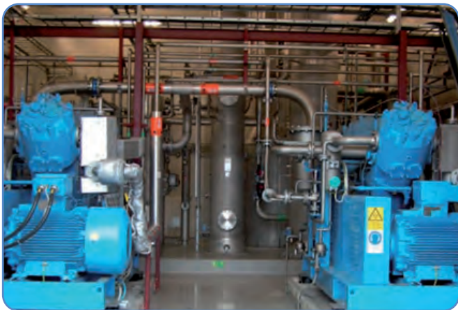
Figure 2 – Upgrading plant with a water scrubber (source: IEA.org)
