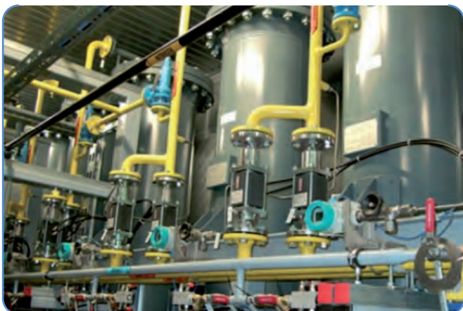
Figure 3 – Upgrading plant using PSA technology (source: IEA.org)
