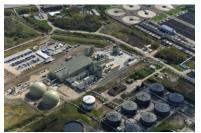
The site is also a major part of UU's sludge treatment and disposal strategy. The site processes 90,000 tonnes per annum (indigenous sludge and from 7 feeder sites), and the thermal hydrolysis and anaerobic digestion plant produce enhanced treated biosolids. CHP engines fuelled by biogas generate electrical energy for the site.
